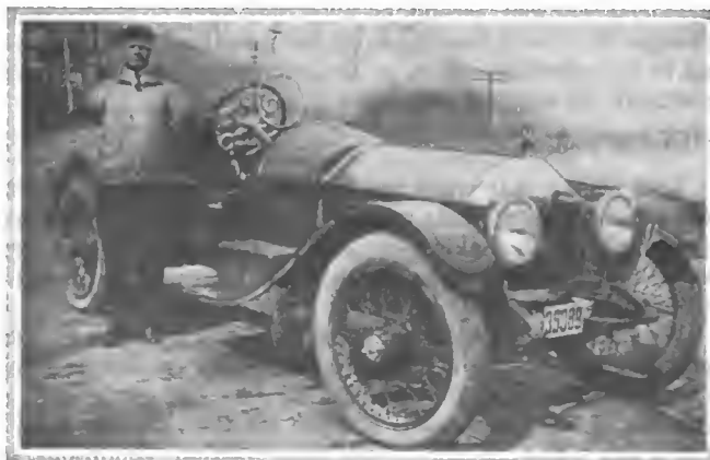
FRANK E. FITHEN of Steubenville, Ohio, who lost both arms in a railroad accident when 9 years old and his six-cylinder Oakland speedster. The gear lever is arranged to be operated by the foot and the steering wheel is fitted with a set of six brass rings forming sockets for Mr. Fithen's arm stubs. These changes enable him to handle the car under all sorts of road and traffic conditions.
